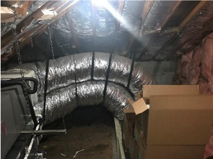
Fiberglass Return Air Ductwork at Mechanical Room
