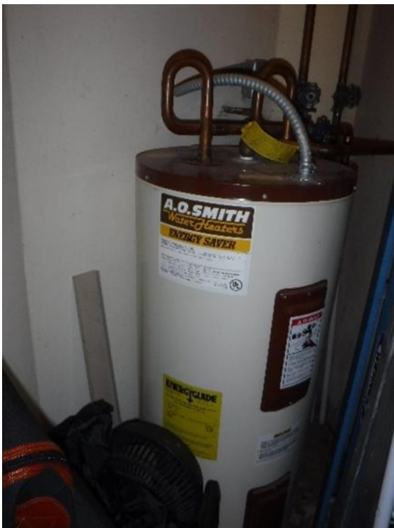
30 Gallon Tank Type Water Heater
