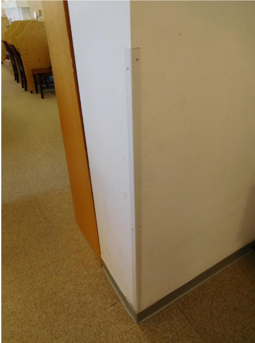
Example of light duty corner guard
