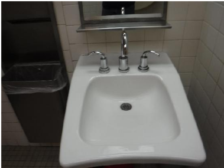
Lobby Women's Restroom Lavatory
