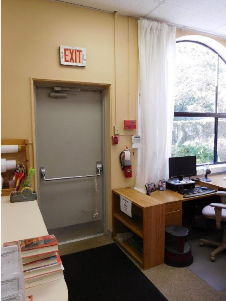
Library Staff Room. Note surface mounted electrical lines.
