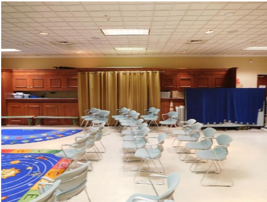
Community Room flooring
