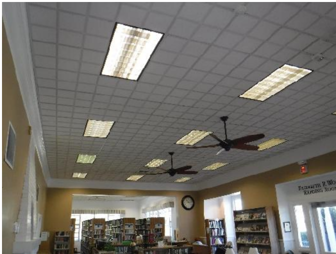
Typical Recessed Lighting Fixtures
