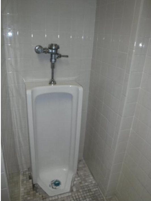
1 st Floor Men’s Restroom Urinal
