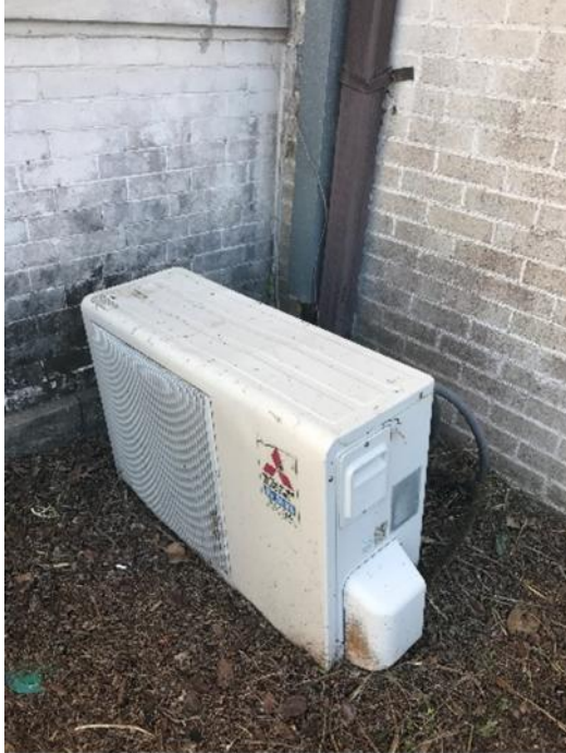
1.0 Ton Condensing Unit
