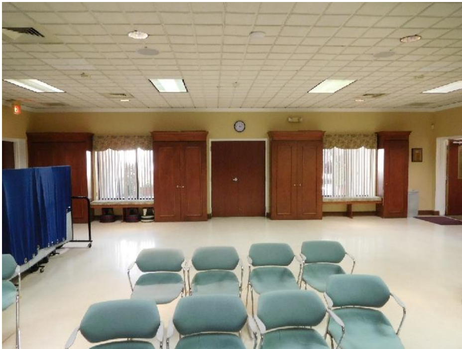
Community Room Ceiling Tiles
