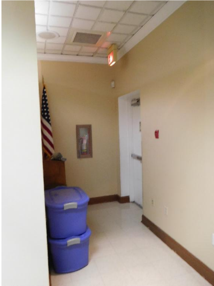
Community Room Egress Exit
