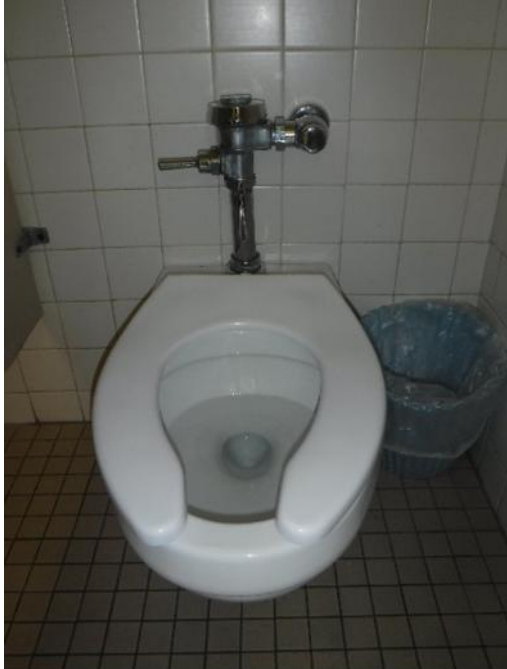
Lobby Women’s Restroom Water Closet
