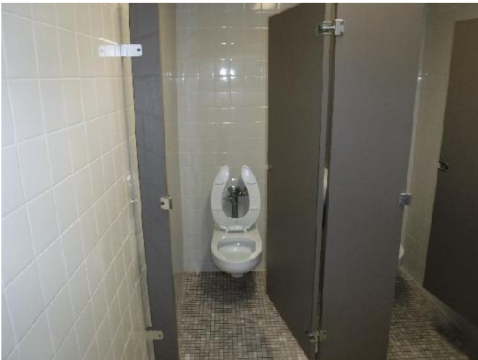
1 st Floor Men’s Restroom Water Closet
