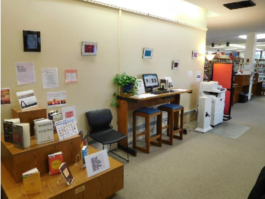
Main Library; Exposed electrical lines.
