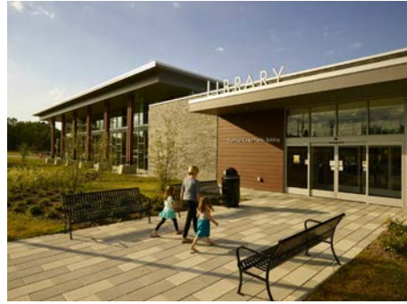
Entry plaza / walkway with benches and automatic bi-parting doors
