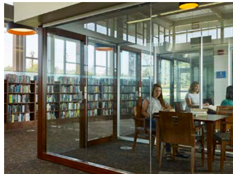
Using demountable partition walls to create study rooms for future flexibility
