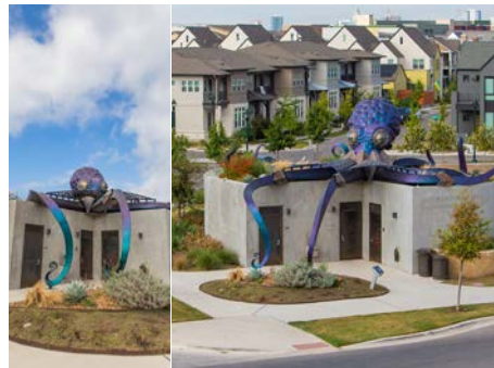
Park restrooms with sculpture
